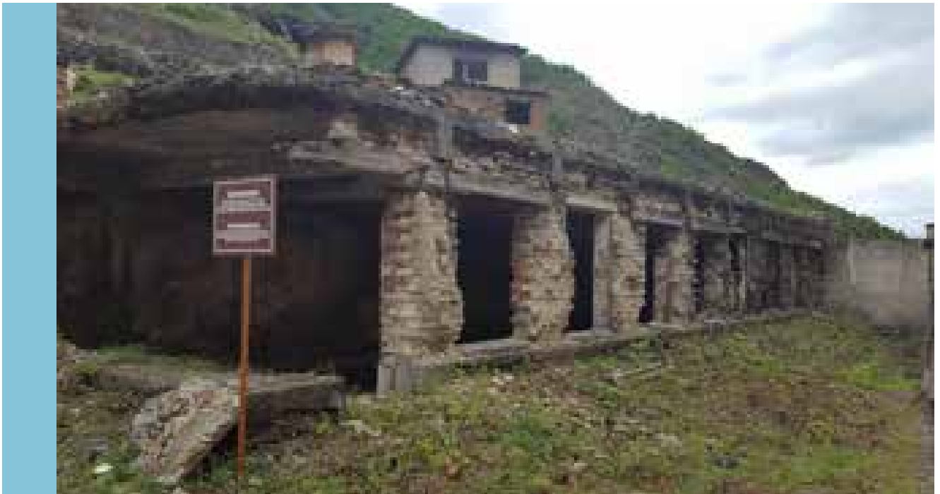
Former Kitchen Hall in Prison of Spaç
